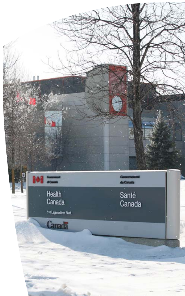
A snowy scene outside the Health Canada building at 510 Lagimodiere Blvd in Winnipeg. Several programs, including the Health Products and Food Program are housed at this location.
